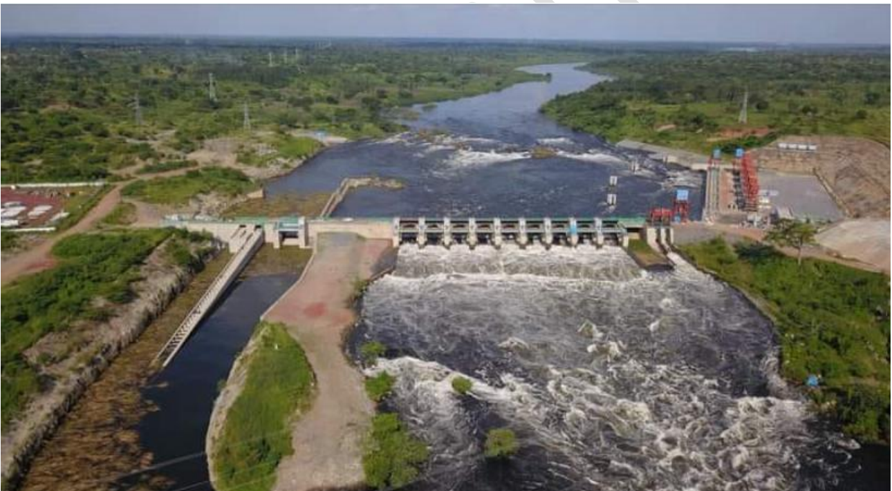
Picture: Karuma hydropower plant in Uganda
